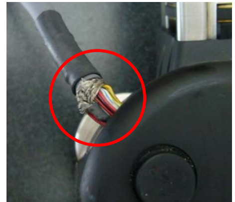
Figure 4.10: Excessive twisting of cable causes damage.
